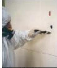
Control measures: shadow vacuuming and using drill cowls as local extraction
