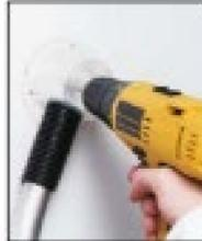
Drill through paste or foam or use a drill cowl and a Class H vacuum cleaner. A hand drill creates less dust. If you have to use an electric drill, put it on the slowest setting.
