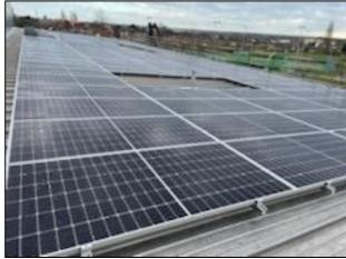
Solar PV panels have been installed at Knighton Library (right), by installer Energy Saving Lighting (ESL). This will help the site to generate their own electricity, reducing their energy use from the grid, thus lowering their carbon footprint.
