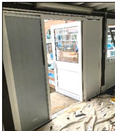
New windows and doors being installed at Caldecote Primary School
