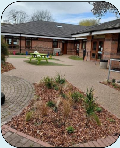
Top row and left - Evington Valley Primary's new raingarden, rainwater planter, water butt and permeable paving.
